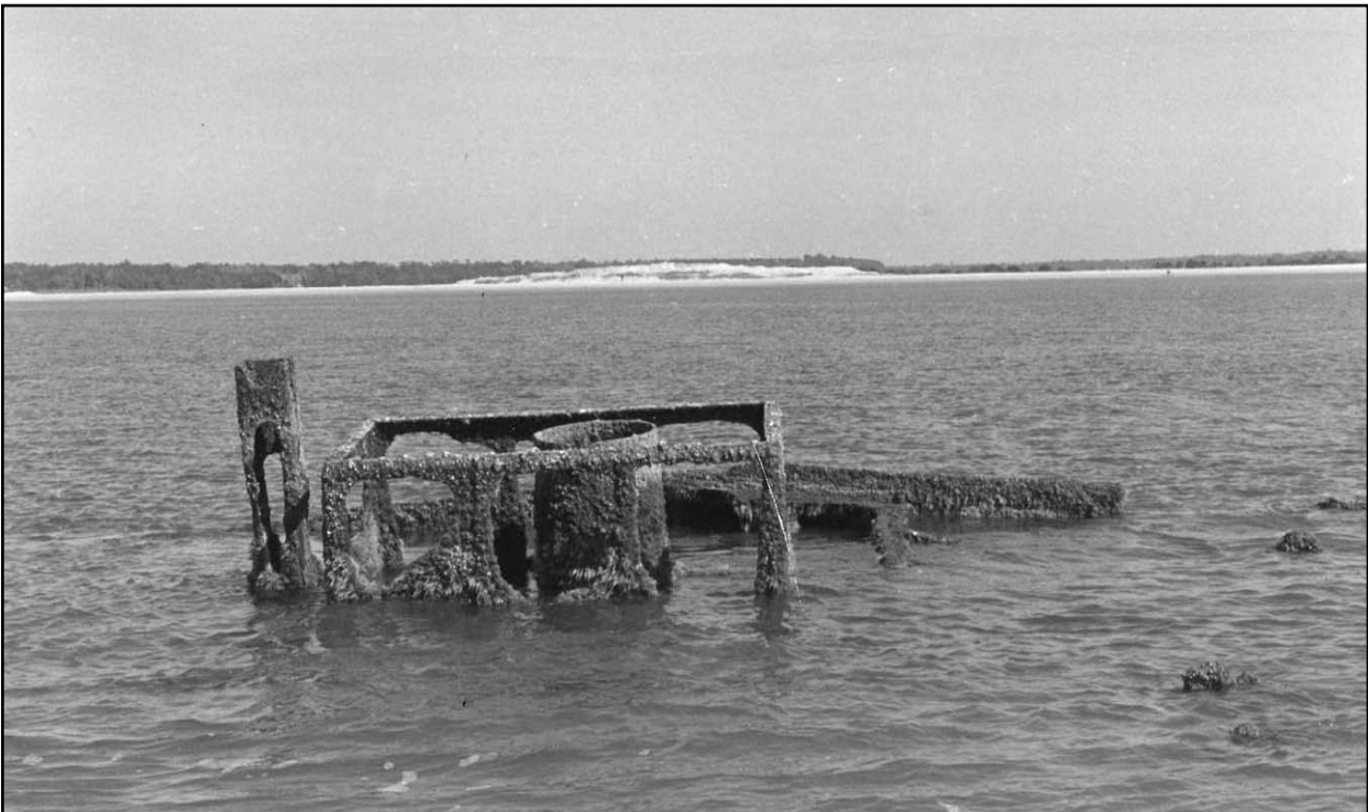
Figure 6: Top of boilers looking east across Lockwoods Folly Inlet from Holden Beach, Site 0001LFI ( Bendigo )
