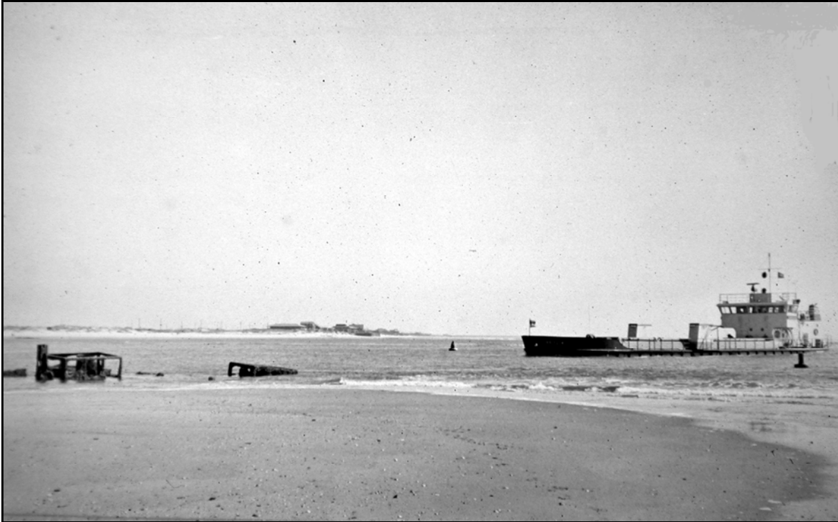
Figure 8: Exposed boilers of the Bendigo (left foreground) and the US Army Corps of Engineers dredge boat, Currituck , Site 0001LFI
