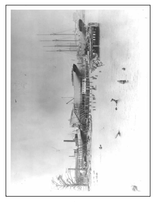
Figure 4. The schooners *Commack* and *Hoppange* under construction at Wilmington Iron Works Shipyard and tugboat hauled out at Stone Marine Railway
